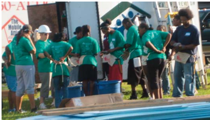
JDCC's Upward Bound students getting ready to begin work on the Habitat for Humanity building project.
